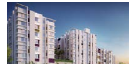
Embee Fortune (Under Construction)
