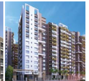
Lumina Apartment (Under Construction)
