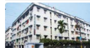
Nil Kamal Apartment (Completed)
